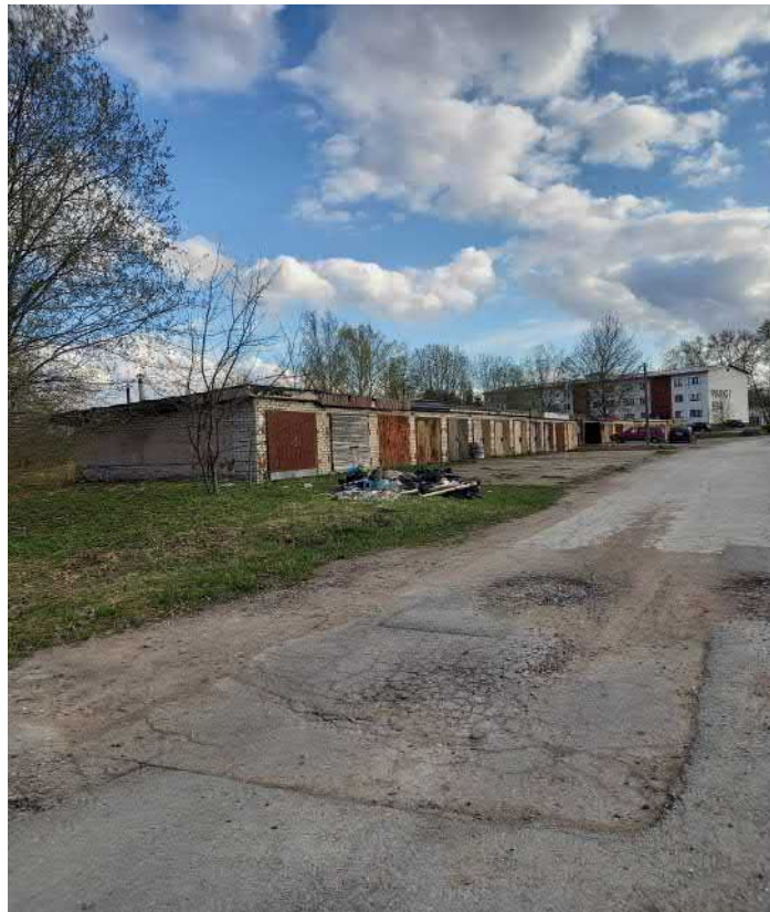
Figure 12. The garages in the area of Malmi-Pargi. (Source: Raagmaa, 2022)
