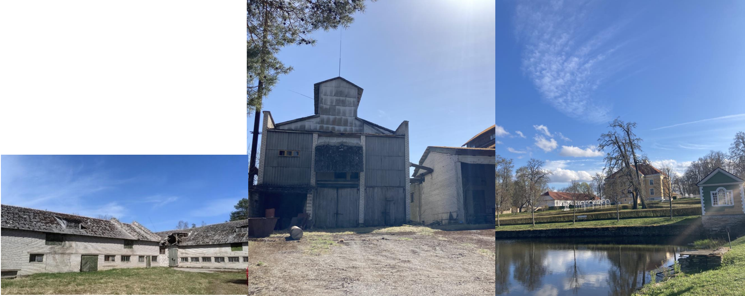
14,15,16 ex. Abandoned cow farm, grain factory, manor with surrounding properties in Palmse
