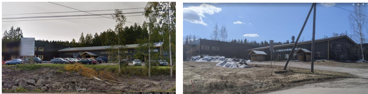
Picture 10 and 11: Industrial building in Savonranta in 2011 (with cars) and 2022 (unused).
