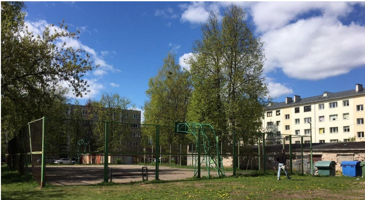
Figure 2318. A dilapidated basketball field in an apartment house area close to the downtown of Daugavpils.
