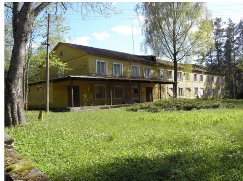
Figure 6. Previous service building 2.0.
