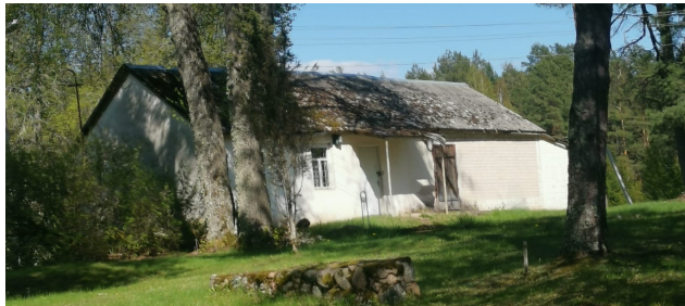
Figure 5. Previous service building.
